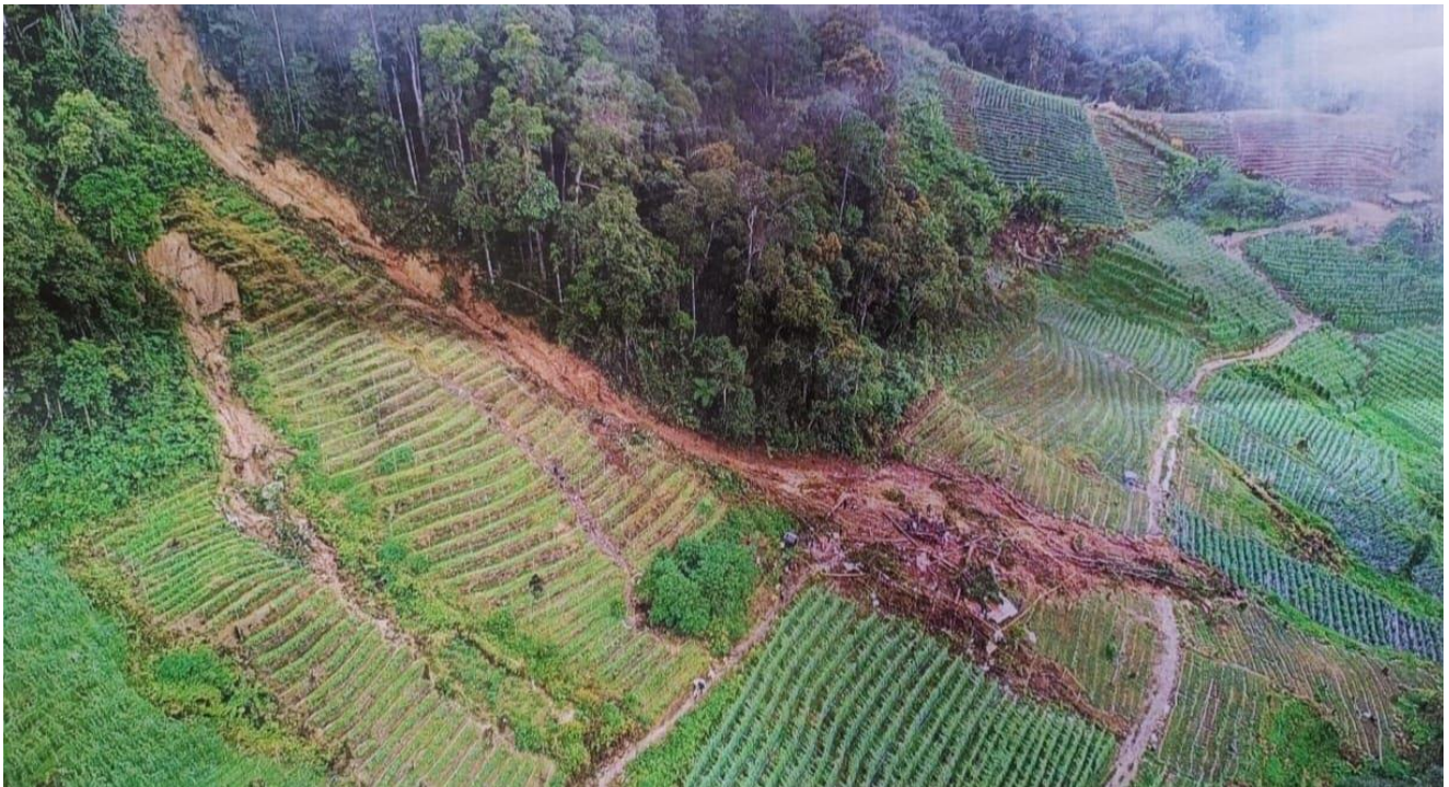
Kejadian tanah runtuh di Cameron Highlands.
