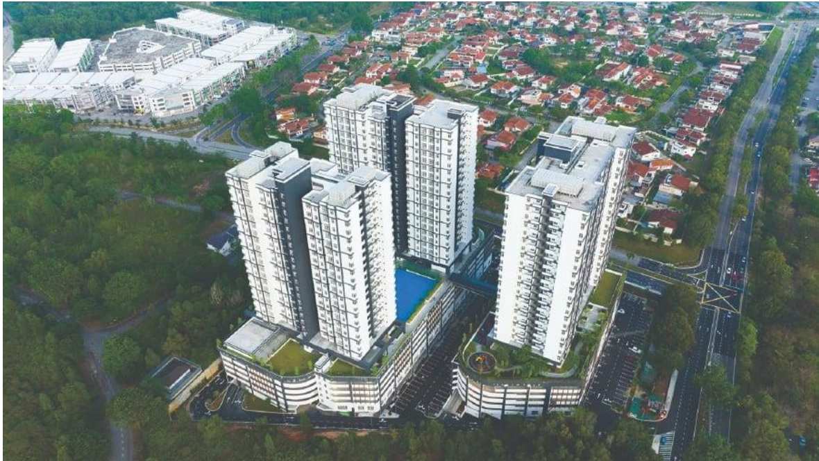
An aerial view of Residensi Bukit Mahkota in Kajang.
